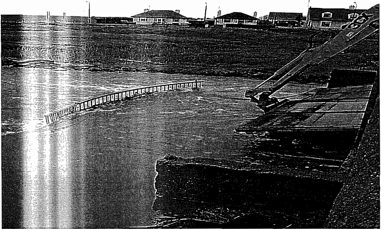
Sluice Gates at Portmarnock Bridge
