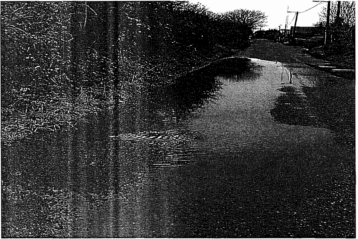
Surcharging of Foul Sewer on Kinsaley Lane
