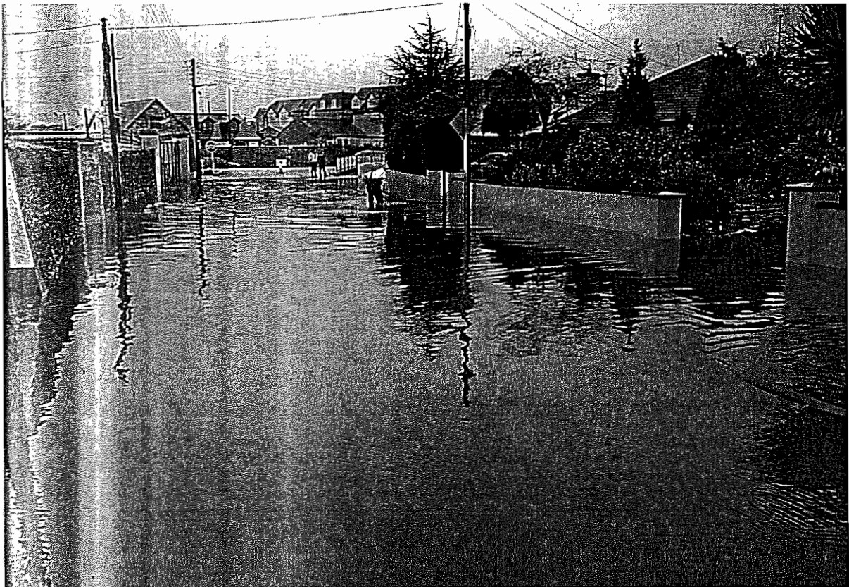
Flooding at North Street/Watery Lane, Swords.
